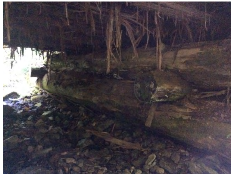
Left Bank Abutment when facing downstream
