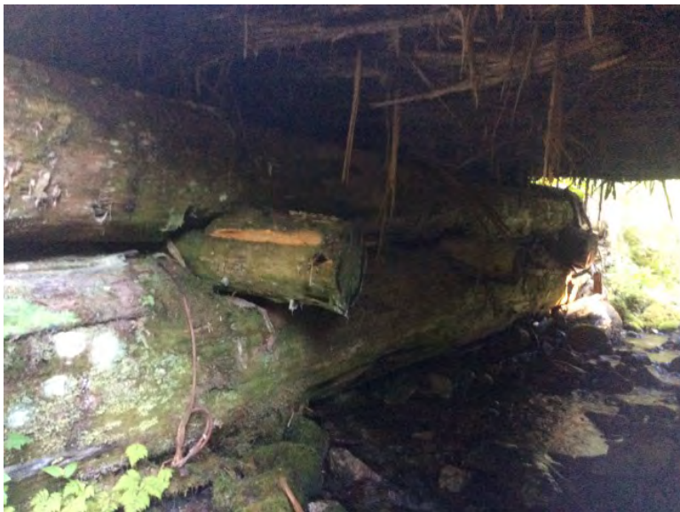
Right Bank Abutment when facing downstream
