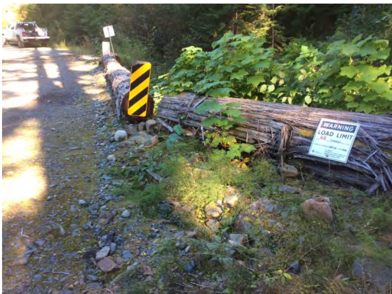
Load Rating Sign
